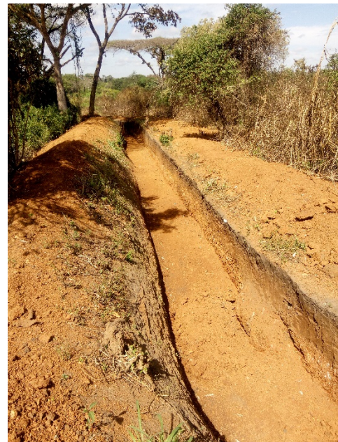
A portion of the 2km trench excavated in Kiyandongo District
